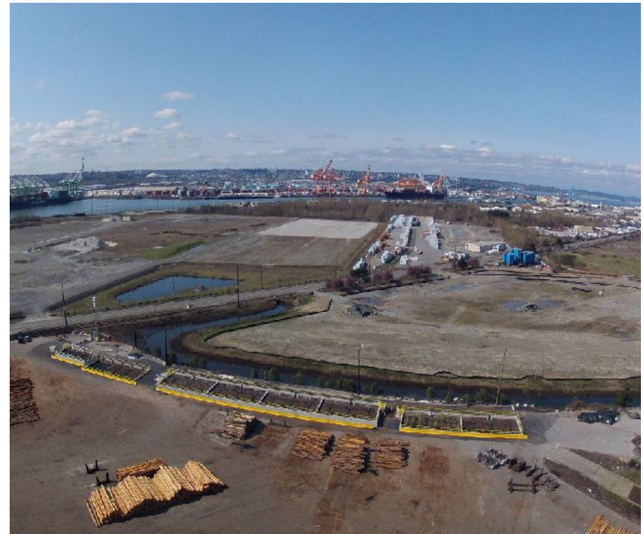
Log yard biofiltration system
